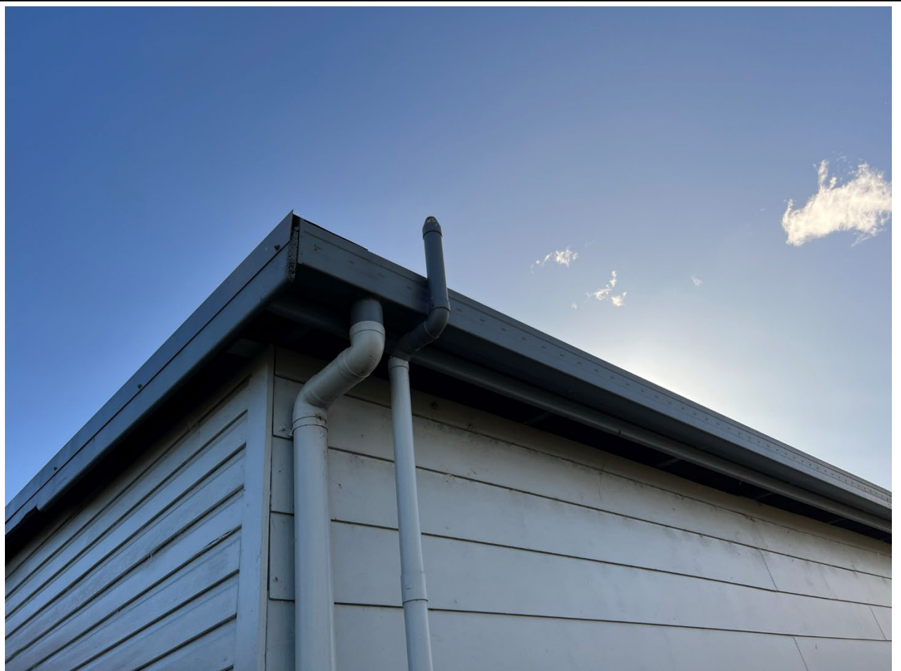
Figure 1 – Existing stormwater drainage
